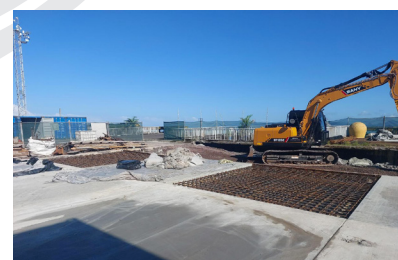
Shed 3 Phase 1 slab pouring progress
