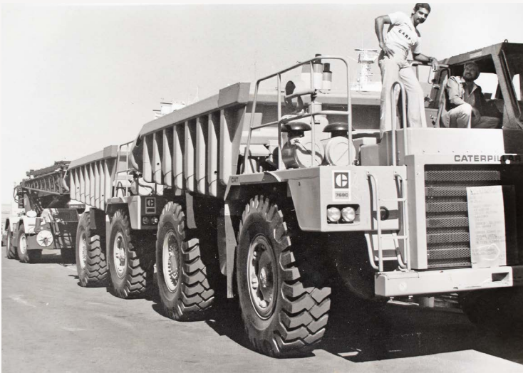
35tonne dump trucks, the first of their kind imported into Fiji for carrying out works at the construction of the Monasavu Hydro plant.
