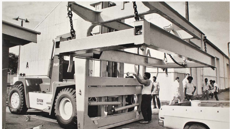
With a lifting capacity of a massive 65,000lb, these were the first of their kind container handling equipment ordered by Ports Authority of Fiji to meet the large number of containers then coming into Fiji.
