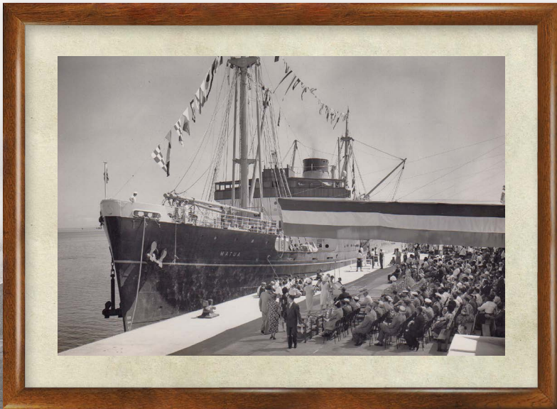
The Union Steamship Company's island vessel MATUA was given the honour of being the first ship alongside the new Suva wharf, The MATUA performed sterling service for Fiji during the war years and had been running regularly to the islands for a quarter of a century.
