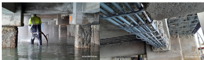
Hydro-demolition works in progress and Queens Wharf Rehabilitation Project-Bay 6 Beam
