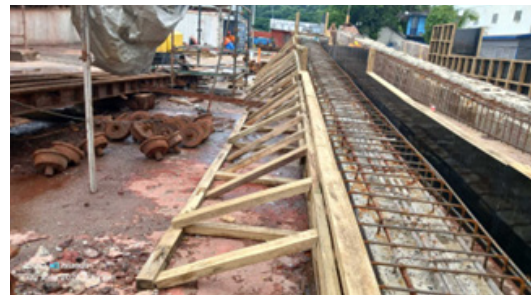
Slipway 500T above water works - Erection of form work
