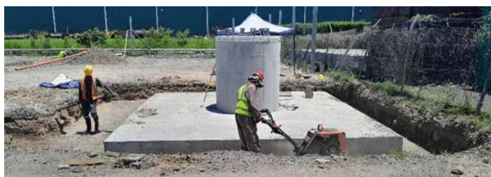
Vibratory compaction around tower light foundations
