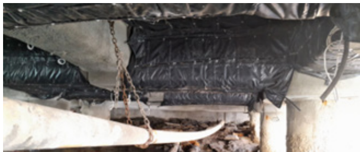
Green Tech Shield Jackets installed at Link Bridge stage 6A
