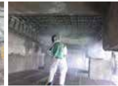
Gunite works to reinstate soffits below Lautoka local wharf
