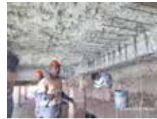
Steel reinstatement works below local wharf
