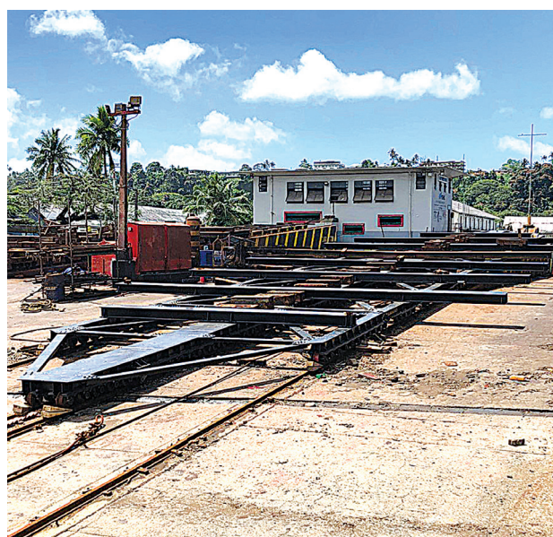
New 500T Cradle Completed in Oct 2020
