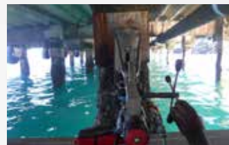
Pile coring under the Levuka wharf deck during the site investigation
